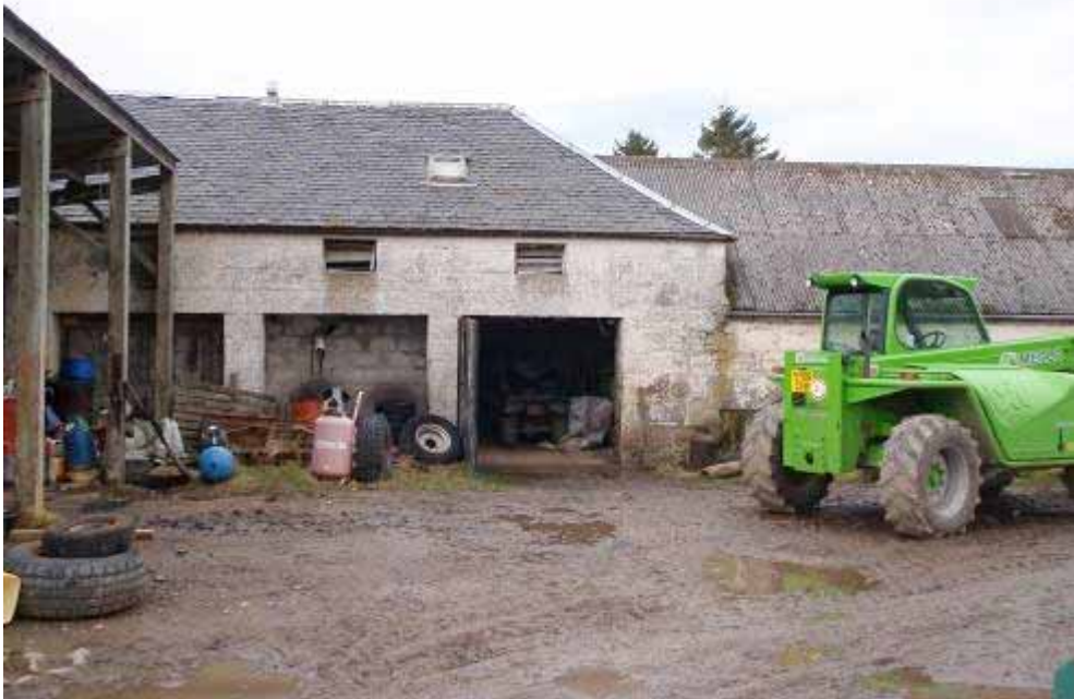
Fig.6-Courtyard View of Steadings
